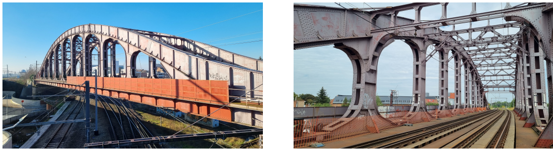
Figure 1: East (left) and south (right) view of the M2.17 railway bridge.
