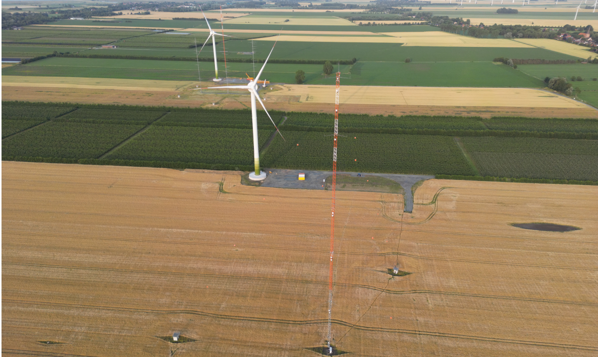
Figure 1: Overview of the WiValdi Research Wind Farm in Krummendeich, Germany. In the foreground is the 150 m mast, followed by the first wind turbine and the mast array. Behind the array is the second wind turbine. At this point (as of January 2025), the experimental turbine is currently under construction.
